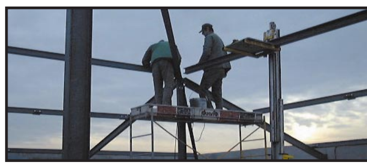
Construction begins on the ORT Montreuil School
