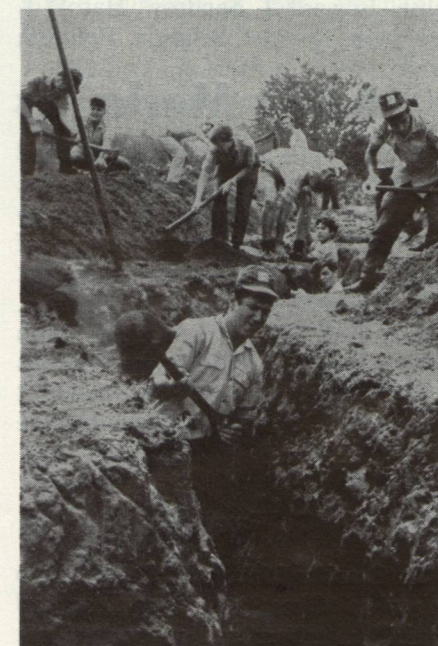
Students dig trenches on school grounds.
