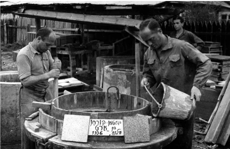
Working with cement at ORT Vilna (Vilnius), 1936.
