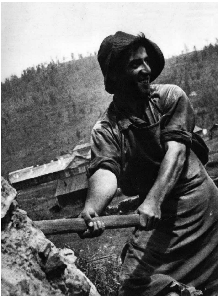
Comrade Torchik, a worker of the lime plant at Londoko, a re-settler from Palestine (undated).
